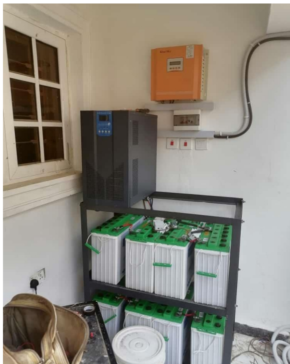
5kva inverter installed @ clinic ICPC hqtrs, Abuja
