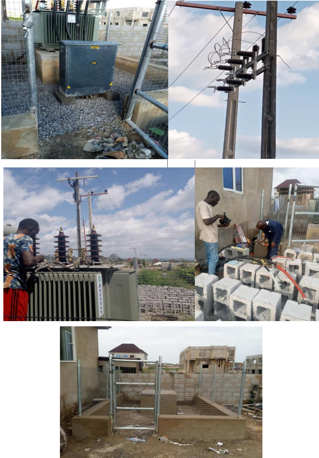
500kva transformer substation @ Wonder Homes estate, Trade more Lugbe FCT - 2020
