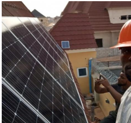
1200w roof-mount solar PV array
