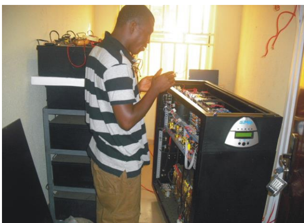
30kva power back up installation
