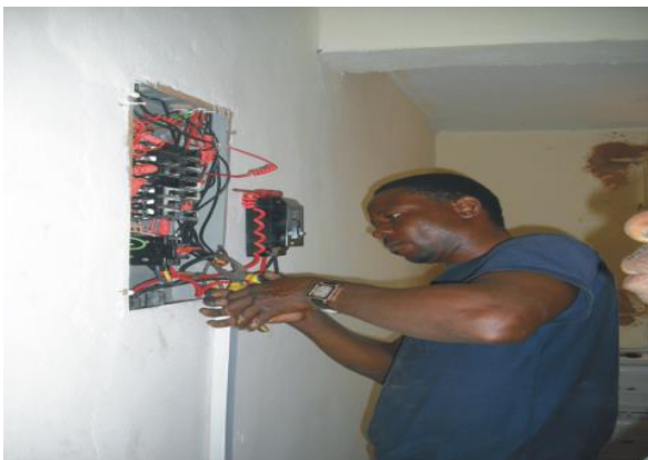
DB installation/Load distribution
