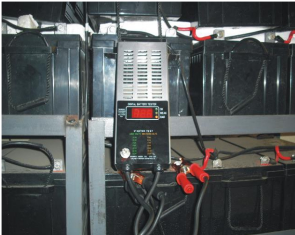
Power bank for inverter system
