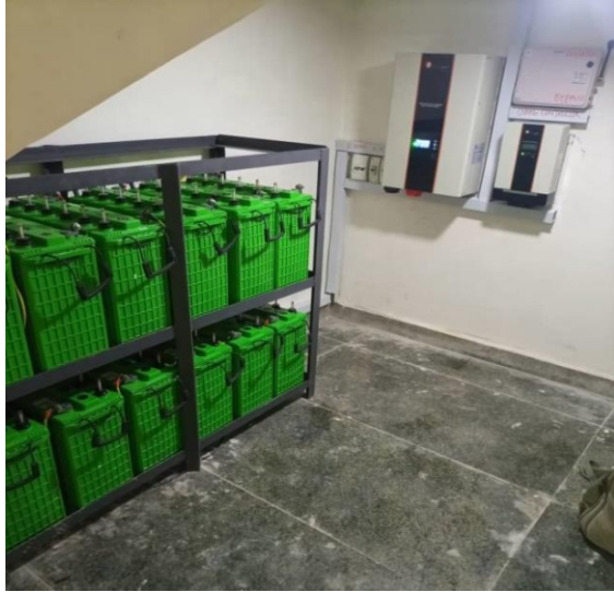
10kva Hybrid solar deployed @ Major Segun Teidi's residence – Sabo Lugbe, airport road Abuja. August 2021
