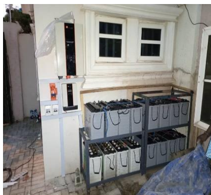
10kva Solar hybrid system deployed @ 3Lions court, Suncity estate, Abuja, 2020
