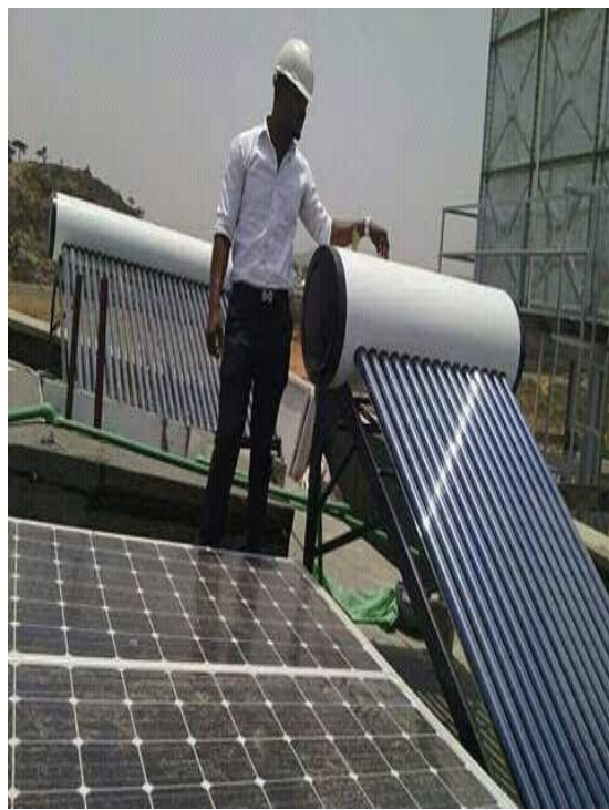
Solar water heater system installed @ Guzape Abuja
